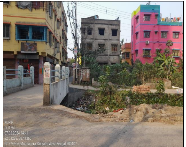
Outfall at Nazirabad(OF13)
